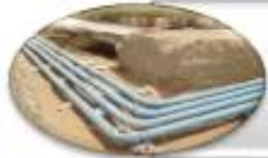
Installation of Underground Water Pipelines
