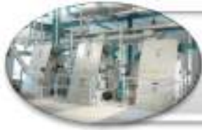
Installation of Coarse/Fine Screens with Screw Conveyor
