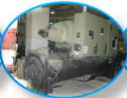
Installation of Chiller
