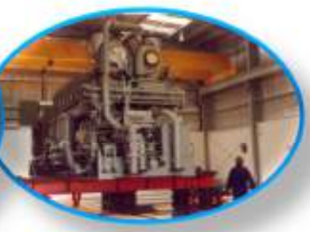
Installation of Generator
